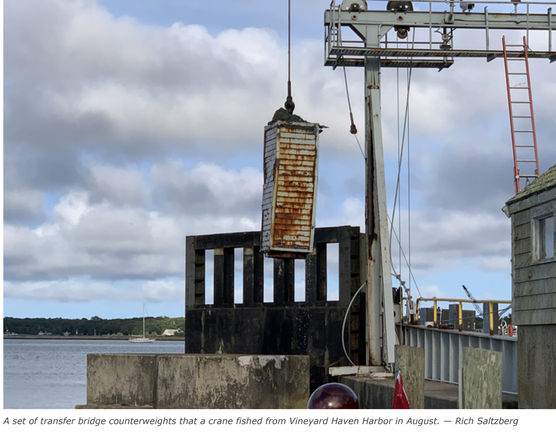
A set of transfer bridge counterweights that a crane fished from Vineyard Haven Harbor in August. — Rich Saltzberg
