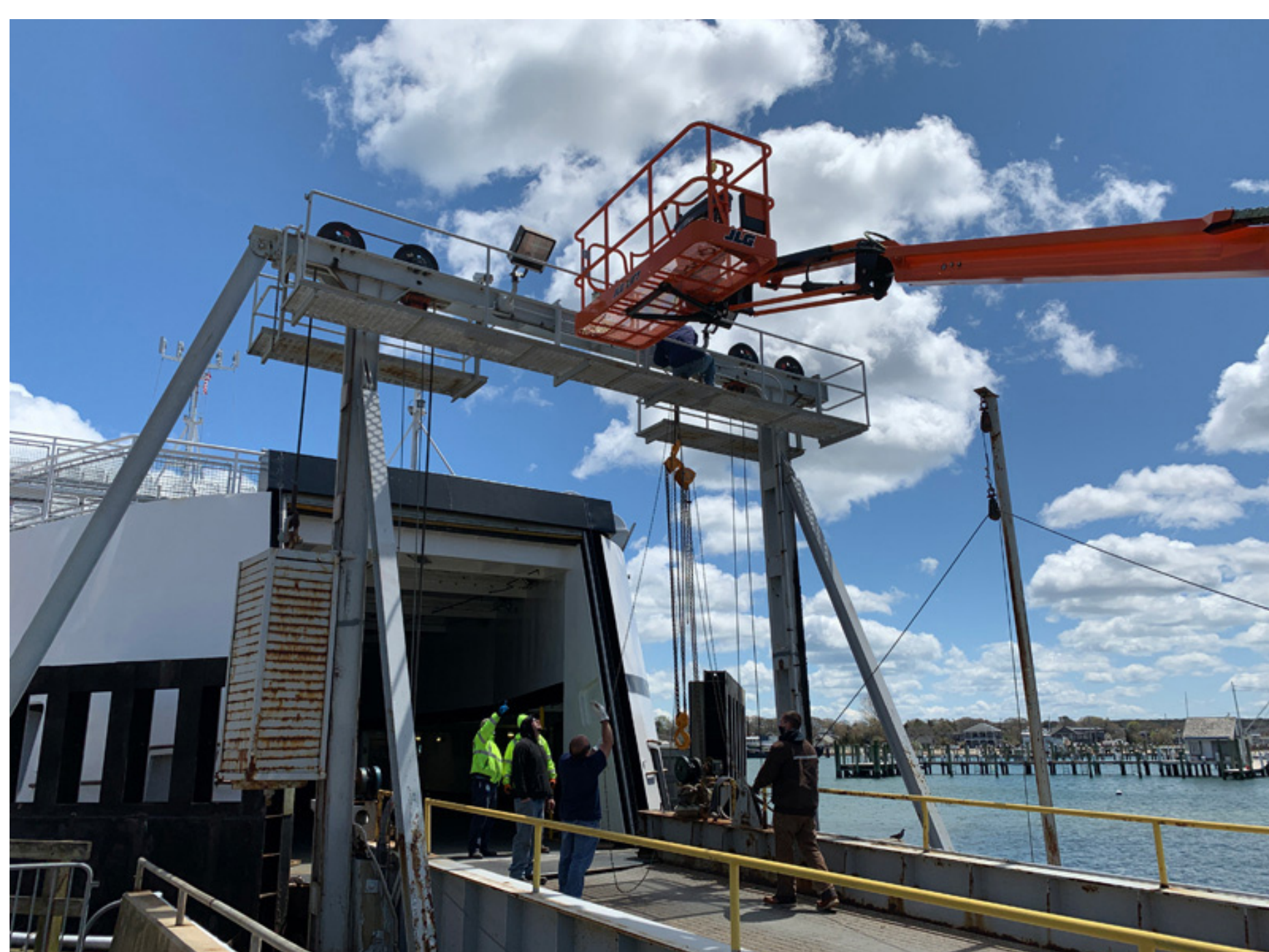
Steamship Authority maintenance and terminal personnel work on May 9, 2020 to repair the Slip 1 transfer bridge in Vineyard Haven after a cable snapped and sent a set of counterweights into Vineyard Haven Harbor. — Rich Saltzberg
